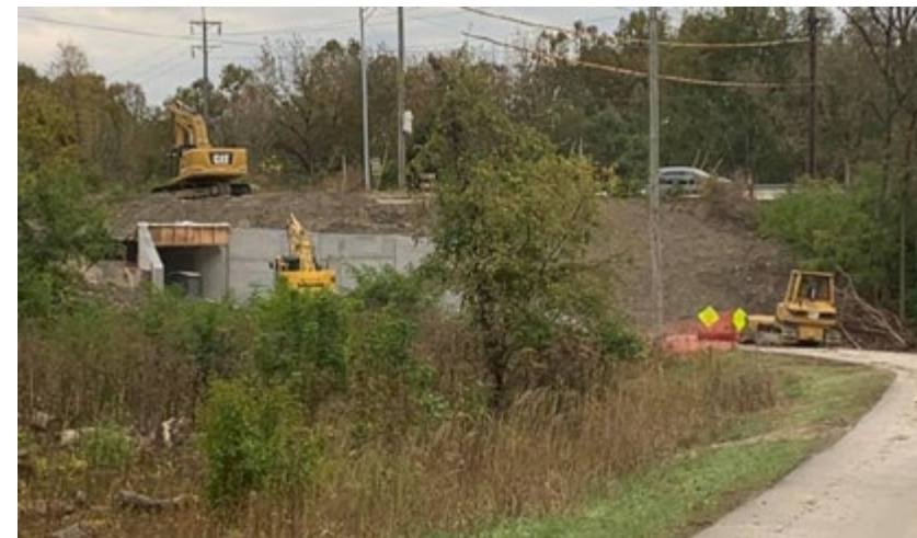
Construction of the Beechmont Connector along the Little Miami Scenic Trail
