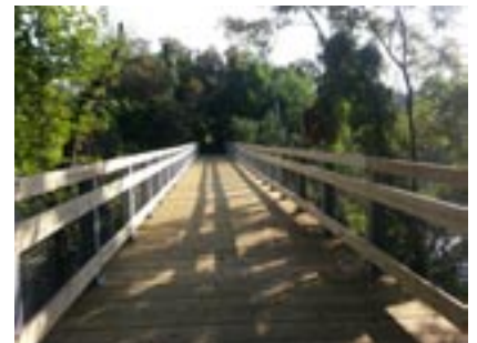
The Galena Brick Trail Bridge
