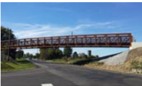
A new bridge on the HOOT, south of Centerburg, Knox County
